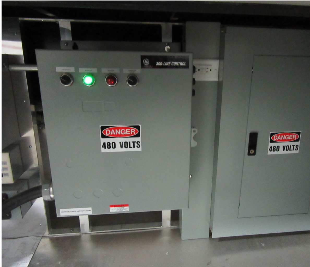
Figure 26: 480V Line Control Box
