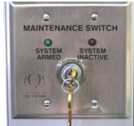
Figure 23: Maintenance Switch
