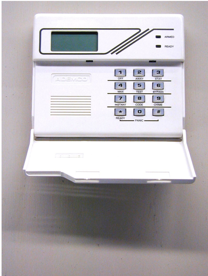
Figure 40: Intrusion Alarm Keypad
