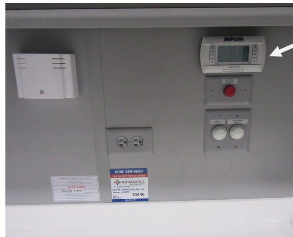
Figure 33: Humidity Controller
