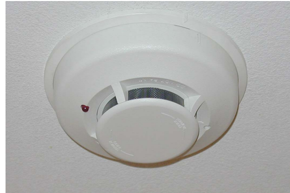
Figure 17: Smoke Detector
