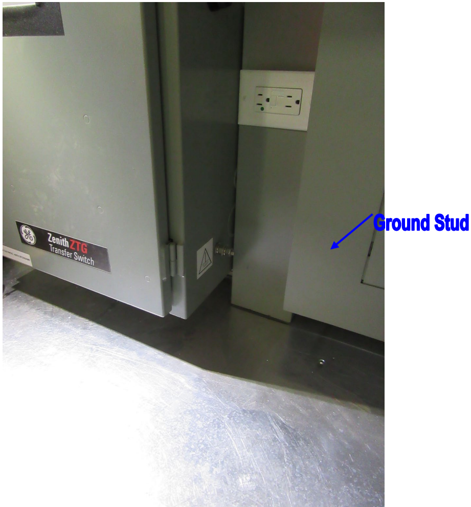
Figure 31: Ground Connection
