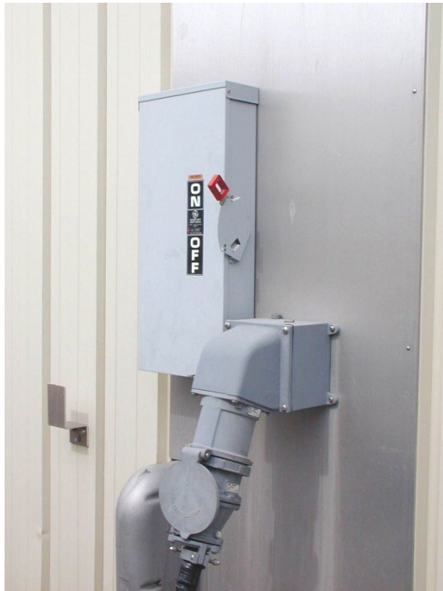
Figure 28: Shore Power Connection
