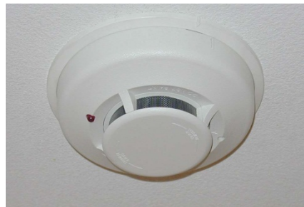
Figure 17: Smoke Detector
