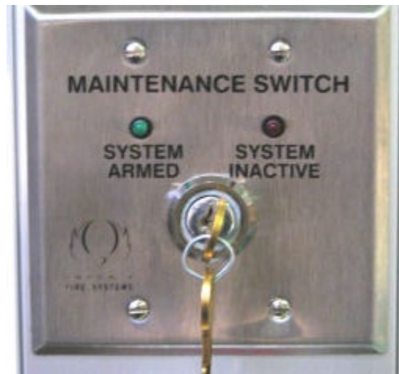
Figure 22: Maintenance Switch
