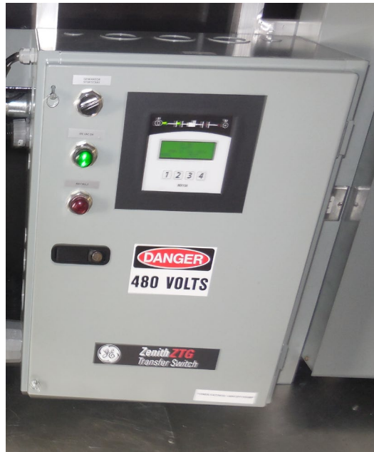
Figure 24: Automatic Transfer
