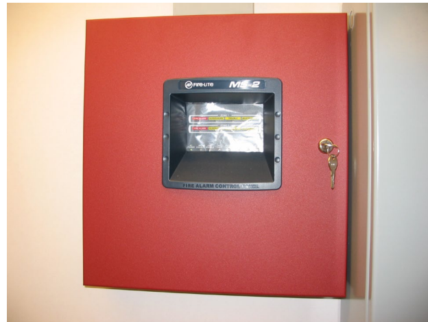
Figure 27: Fire Alarm Control Panel
