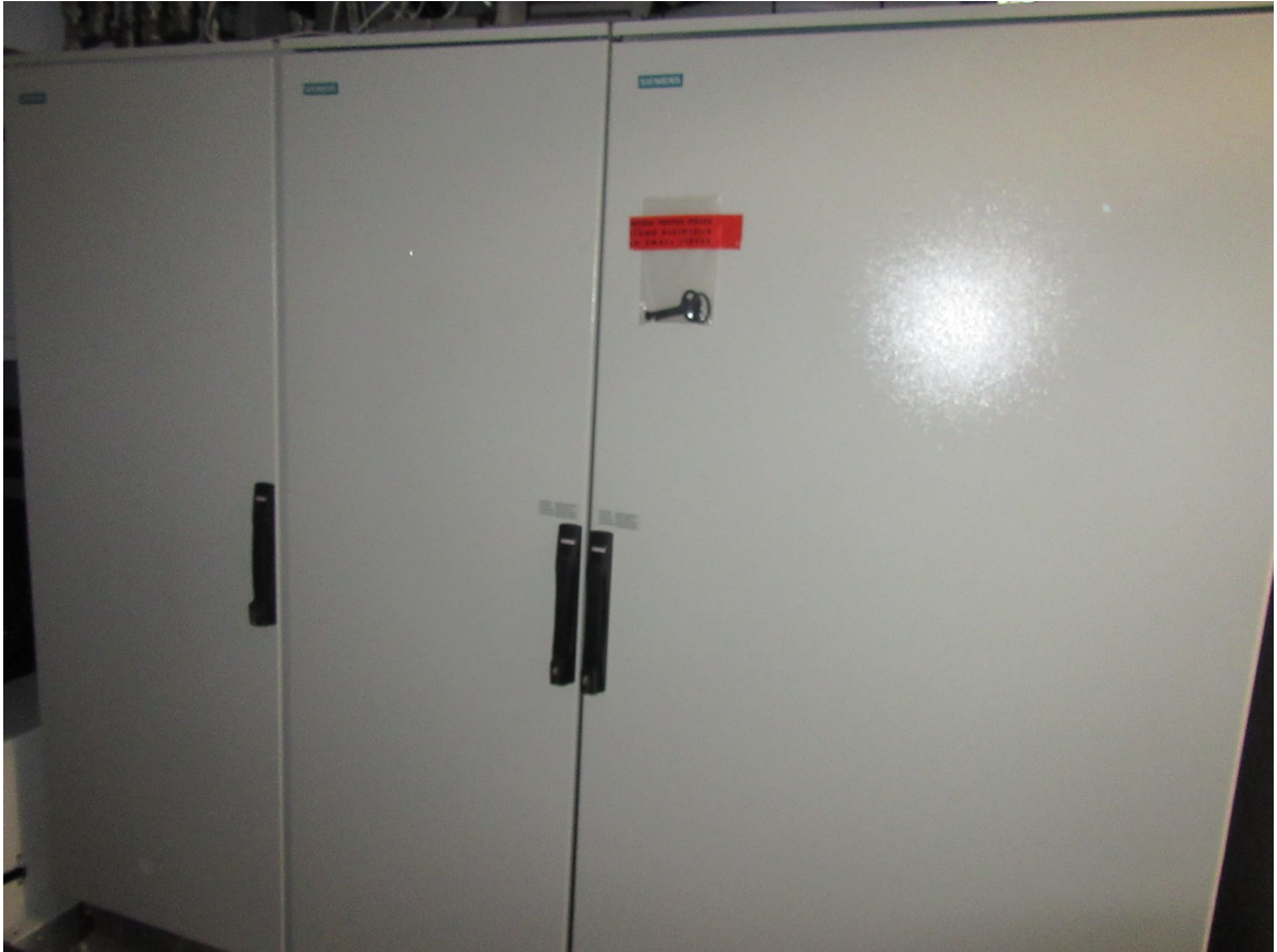
Figure 6: Cryogen Compressor Cabinet
