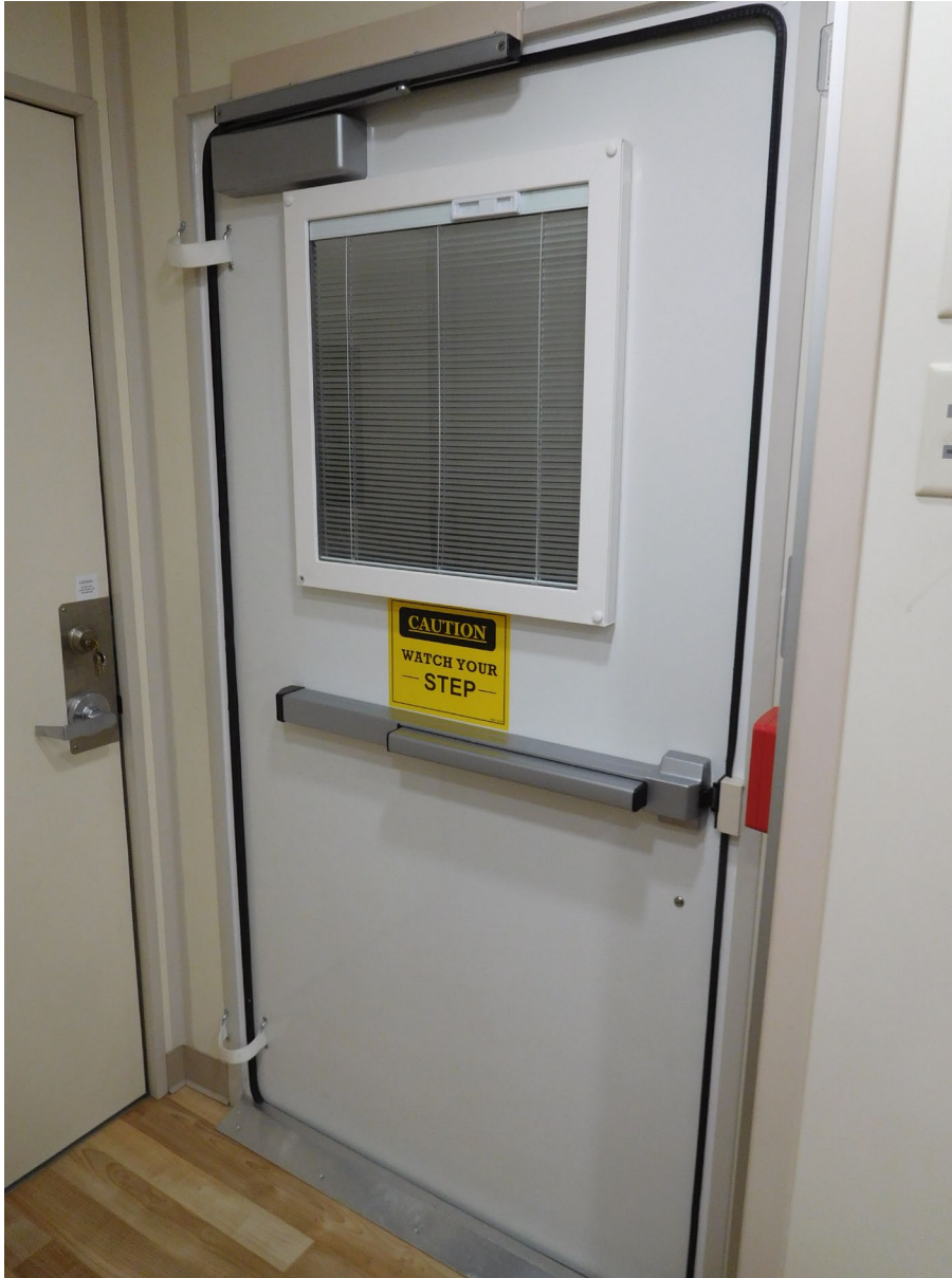
Figure 9: Exterior Staff Door
