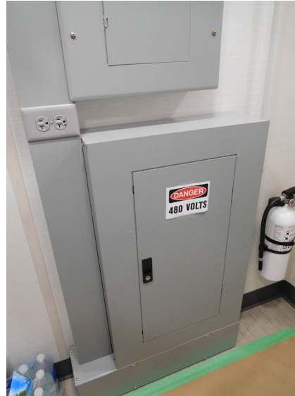
Figure 36: 480V AC Electrical Panel
