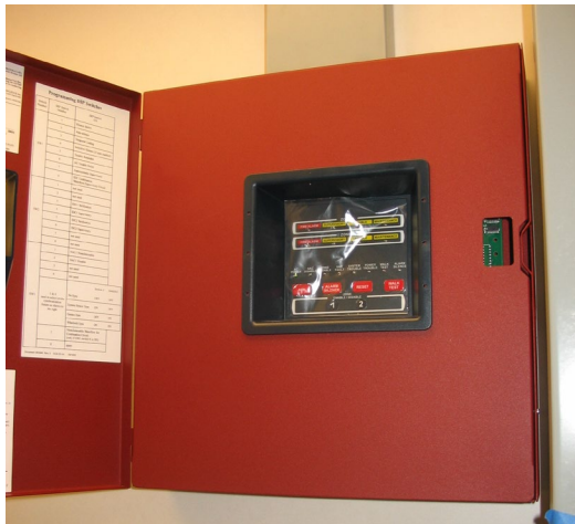
Figure 27: Fire Alarm Control Panel
