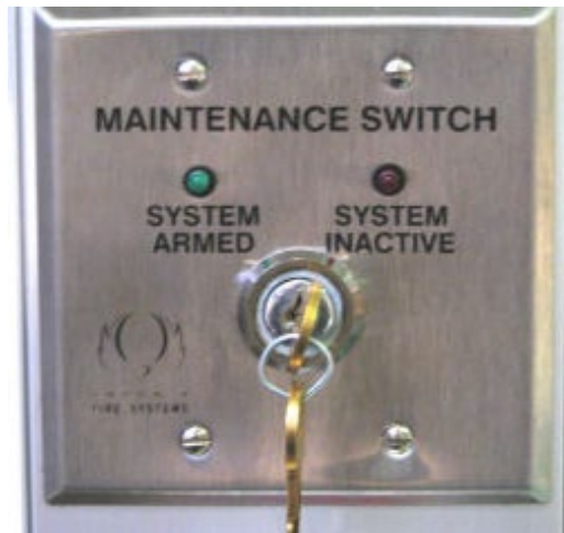
Figure 32: Maintenance Switch
