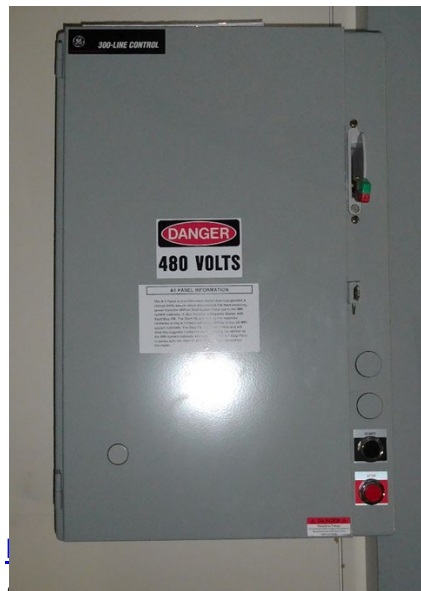
Figure 36: 480V AC Electrical Panel
