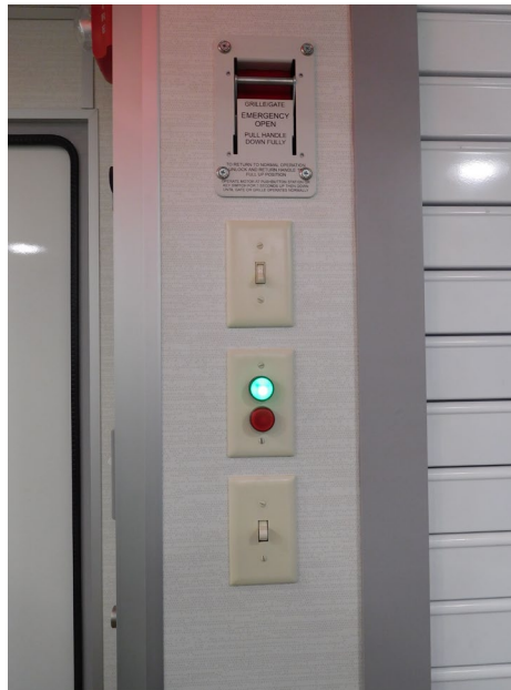
Figure 33: Roll Door Emergency Release
