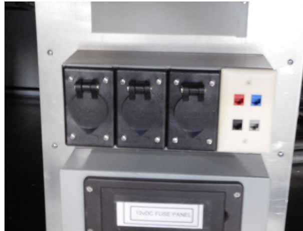
Figure 17: Phone & Data Line Connections
