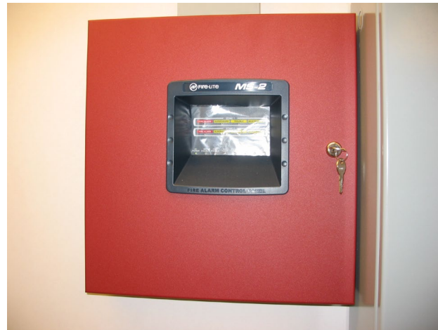
Figure 27: Fire Alarm Control Panel
