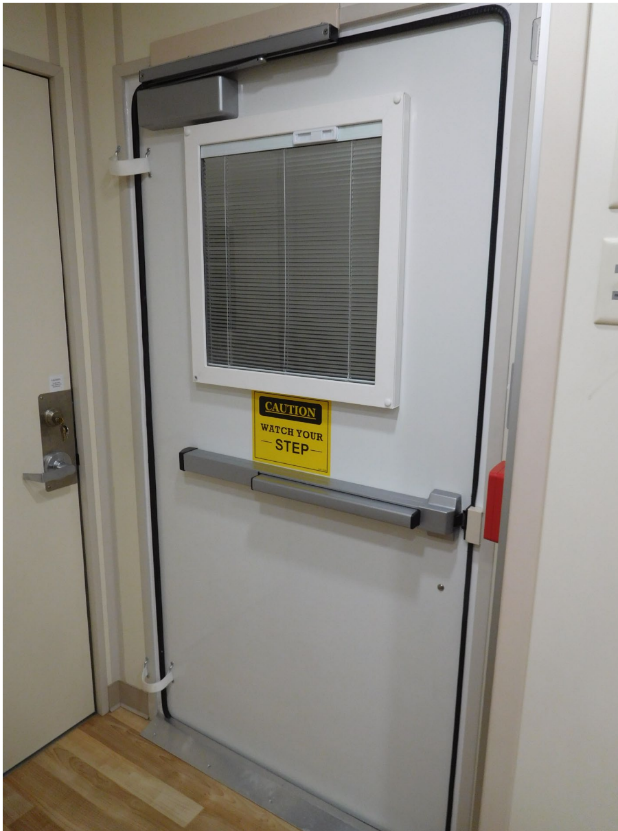
Figure 9: Exterior Staff Door
