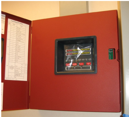
Figure 27: Fire Alarm Control Panel
