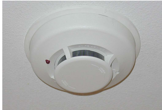
Figure 26: Smoke Detector
