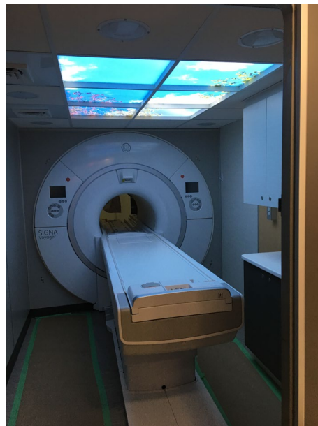
Figure 61: Scan Room Lighting
