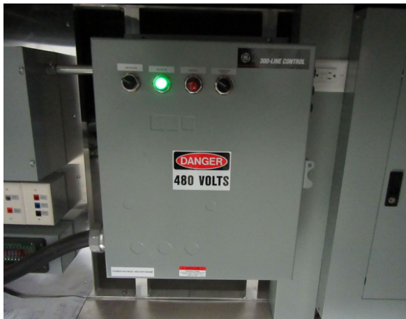
Figure 28: 480V AC Electrical Panel (underbody)
