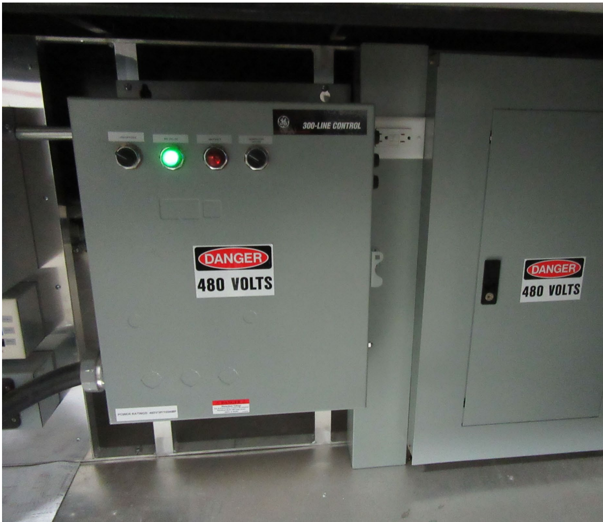
Figure 26: 480V Line Control Box
