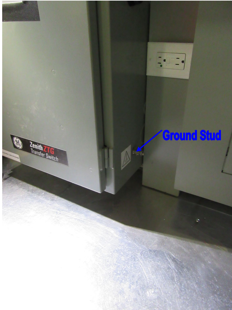
Figure 31: Ground Connection
