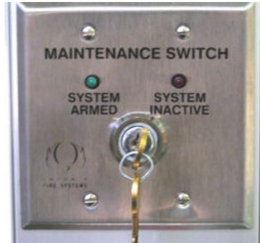
Figure 23: Maintenance Switch
