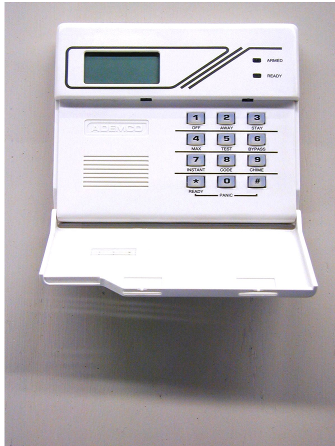
Figure 40: Intrusion Alarm Keypad
