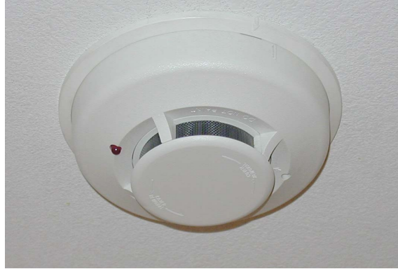
Figure 17: Smoke Detector
