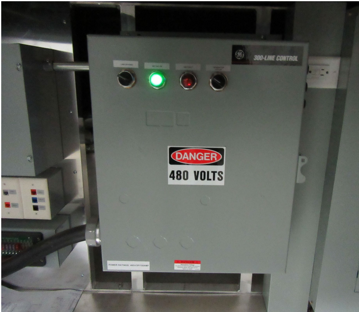
Figure 27: 480V AC Line Control Box
