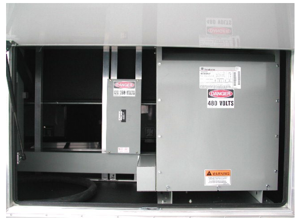
Figure 28: 480V AC Electrical Panel (underbody)
