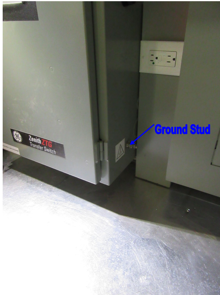
Figure 31: Ground Connection
