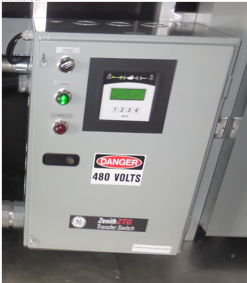
Figure 27: 480V AC ATS and Phase Power Monitor
