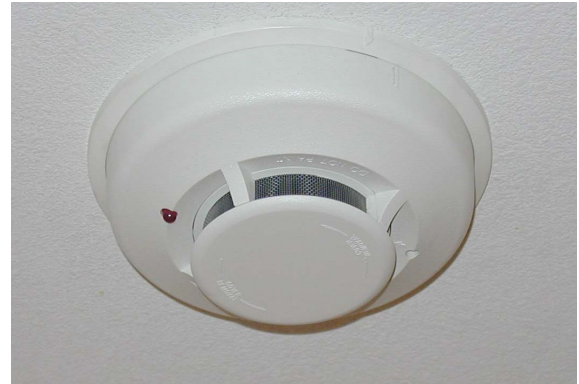
Figure 17: Smoke Detector
