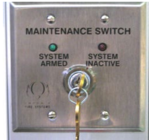
Figure 23: Maintenance Switch
