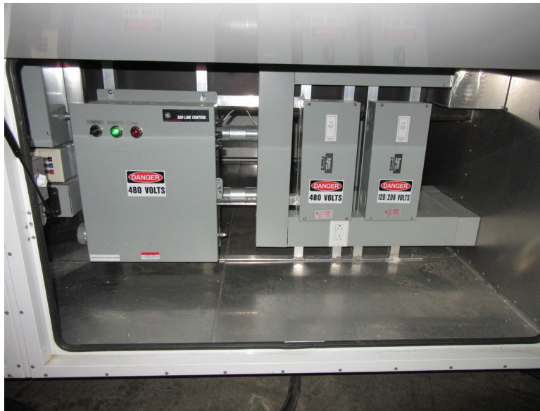
Figure 26: 480V AC Line Control and Phase Power Monitor
