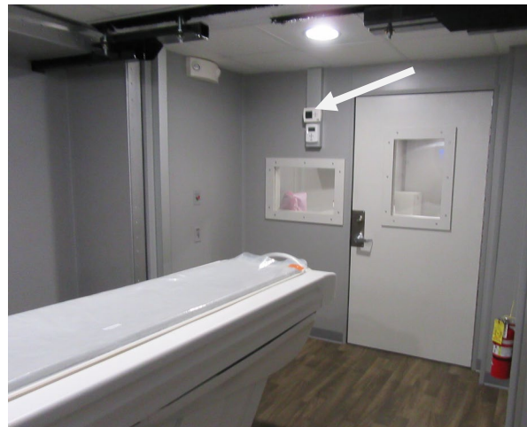
Figure 33: Humidity Controller
