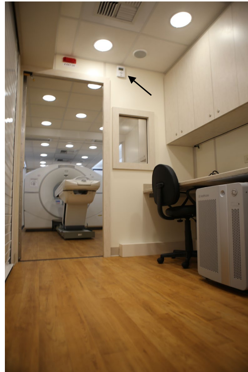
Control Room/Hot Lab Control
