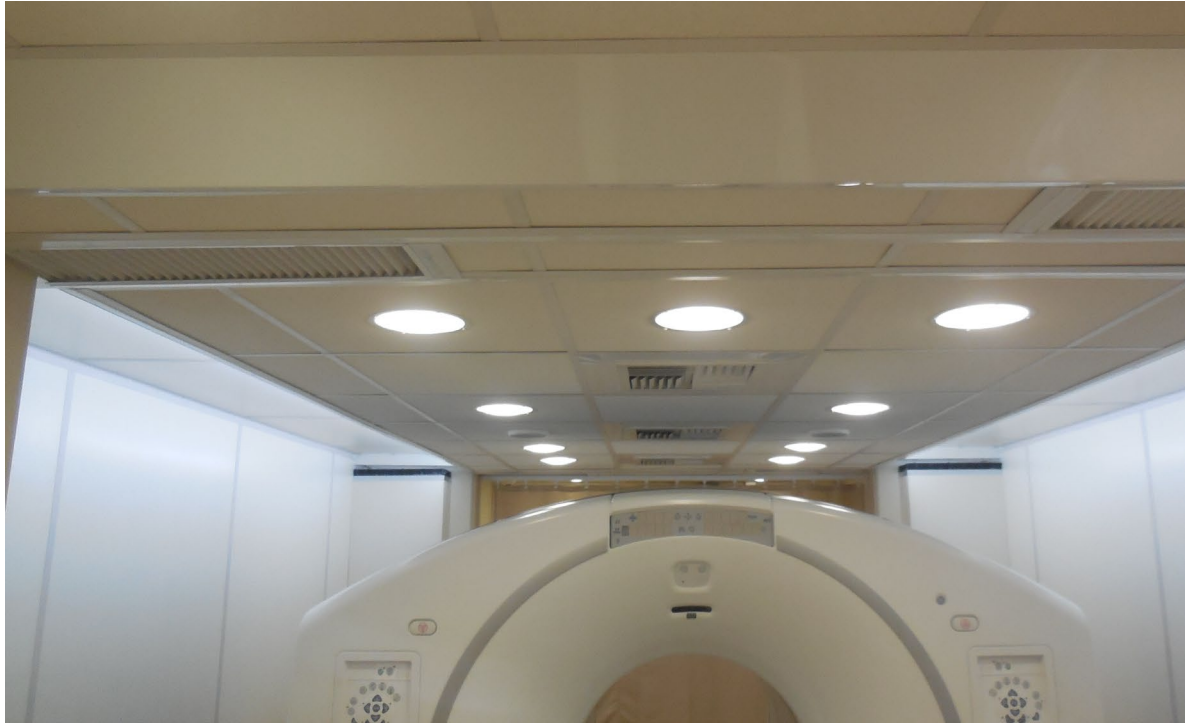
Figure 42: Gantry Room Overall Lighting
