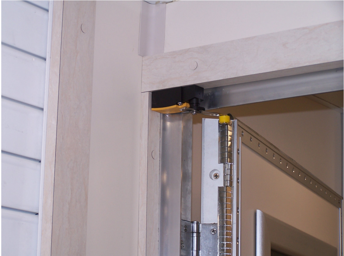
Close up of RF door trim
