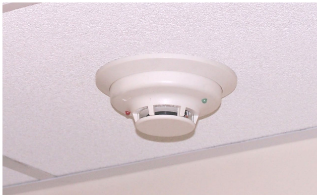
Figure 22: Smoke Detector
