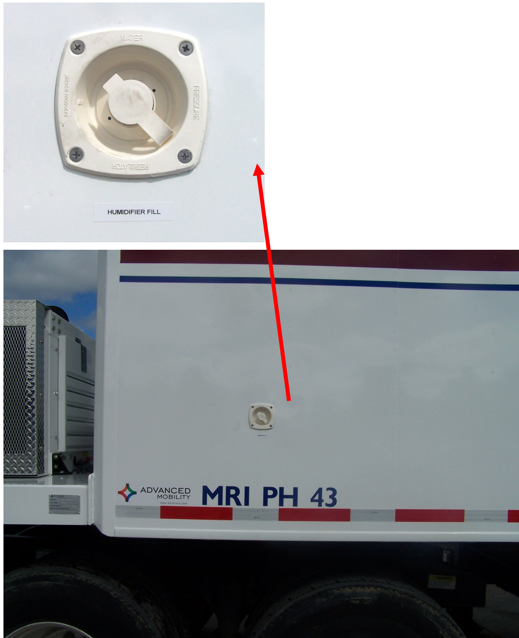
Figure 18: Fresh water Connection
