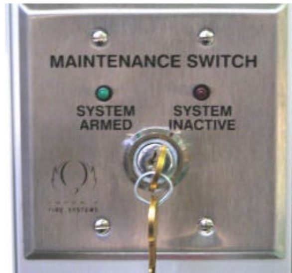
Figure 28: Maintenance Switch
