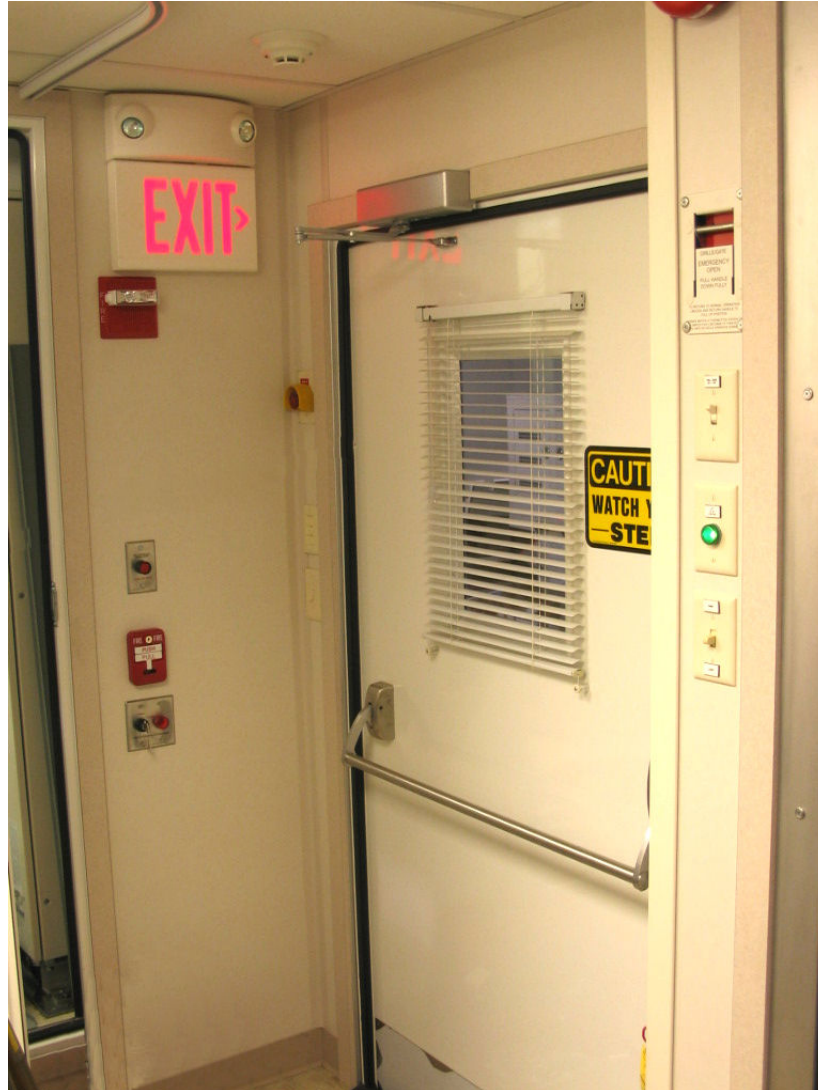
Figure 8: Exterior Staff Door
