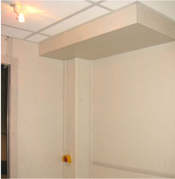
Figure 17: Magnet Room E-Stop & Quench Buttons
