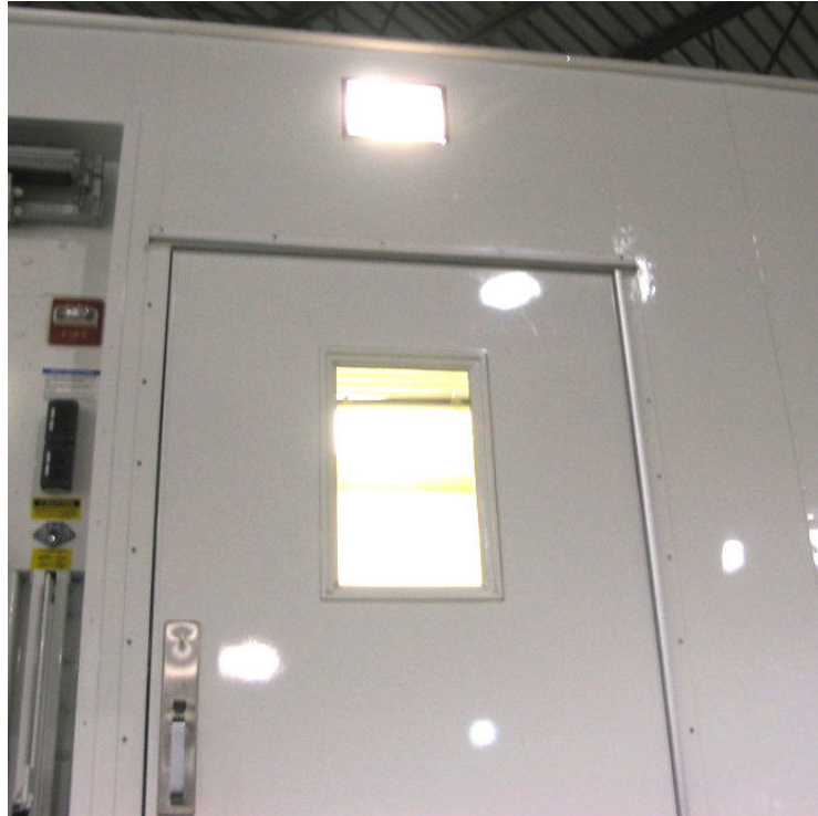
Figure 55: Staff Door Lighting
