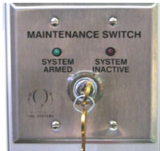
Figure 31: Maintenance Switch
