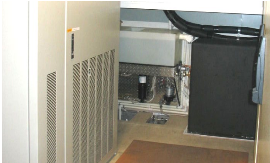
Figure 43: Humidifier Tank
