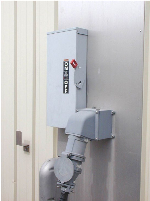
Figure 26: Shore Power Connection
